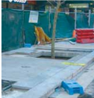
Construction of a planter tree
