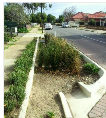
Figure 2-3: A bioretention basin
